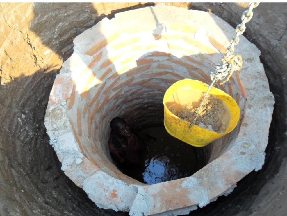
Our collective support of £3,131.76 has funded the labour costs of digging and constructing the 5 new wells, along with the cement, brickforce wire and winding systems. The community, in line with our 'hand up' self-help approach, hand-made the bricks themselves, along with collecting the sand from a neighbouring dry river bed.
