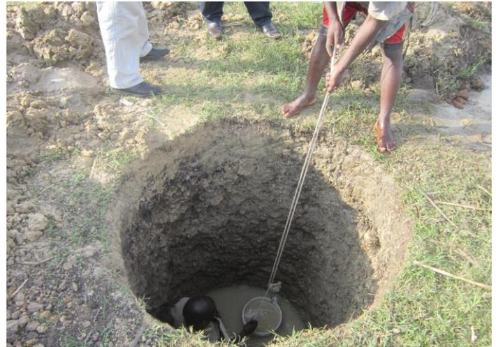
The 6 wells have been built in **Nabirye, Bukona 1, Bukona 2, Nakilurwe, Nawangingi 1 and Nawangingi 2** villages and vary in depth from 25 to 70ft depending on the water table in each location. The excavation was carried out by hand so this was really physical work!
