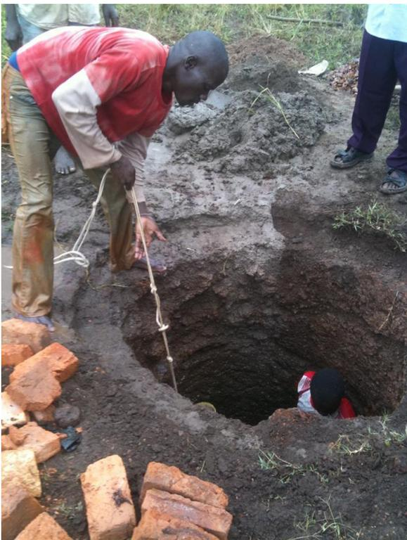
The Busoga wells are different to our Zambian wells, as they incorporate hand pumps via a piping mechanism that draws water up from the bottom of each well. This means that these wells are capped (closed off), reducing the risk of contamination. It also makes it easier to draw water.
